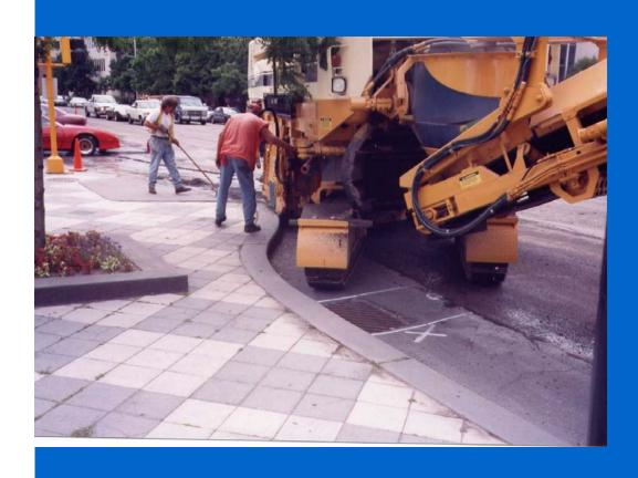
The PR-860 has the power, versatility and maneuverability to take on full- or half-lane work milling to a depth of 12 inches at a maximum width of 84 3/4 inches.
