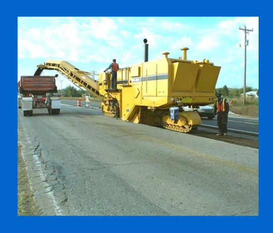
A three-track stance gives the PR-800-7 all the maneuverability and traction needed for big jobs. It also cuts the mill's turning radius and helps the operator steer around obstacles more easily.
