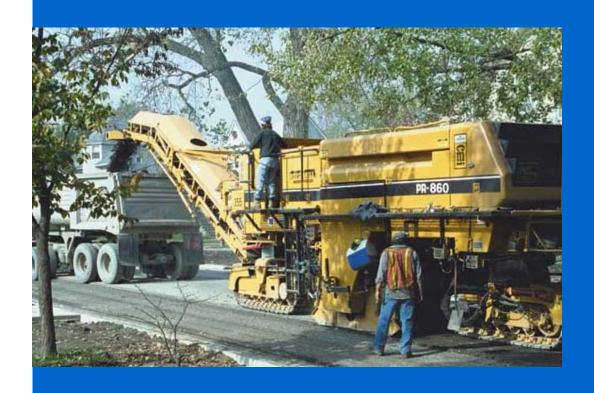
The low-rise PR-860 slips under structures and trees on tight city jobs to let crews work efficiently. Track drive helps an operator steer around ground-level obstacles that could slow the progress of other large profilers.
